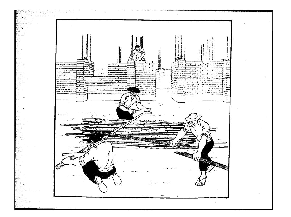
In this drawing, the men are placing the collar beam on the wall.
