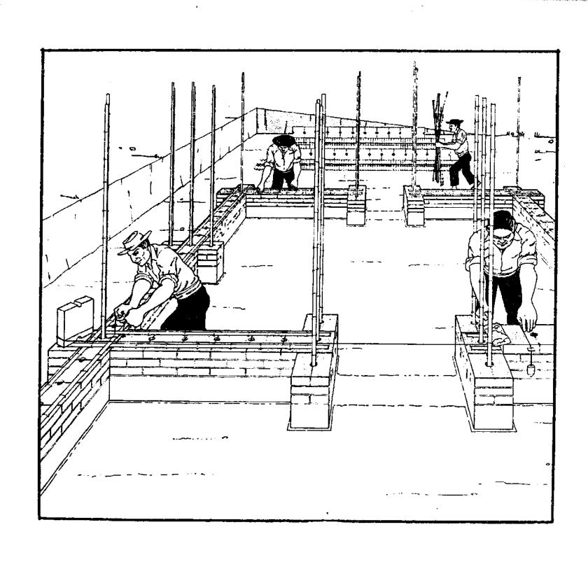
In this picture, the <u>maestro</u> is putting the next layer of adobe over the cane reinforcing. He has checked the position of each adobe to make sure it is level.
