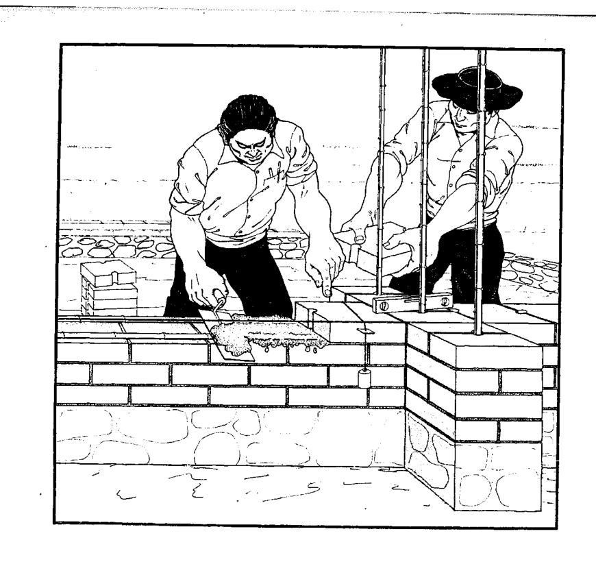
In this drawing, the wall is almost completed and only three or four more layers of adobe are needed. The <u>maestro</u> and his helper are tying wire to one of the canes used as vertical reinforcement. As the last layers of adobe are put on the wall, the free end of the wire will pass up through the hole with the cane. After the last level of adobe has been laid, the wire will be used to attach the collar beam (<u>viga collar</u>).
