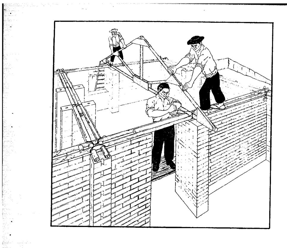
In this drawing, the trusses have been placed on top of the wall.
