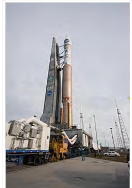
Several lightning protection masts can be seen in the background of this photo of a rocket launch site.
