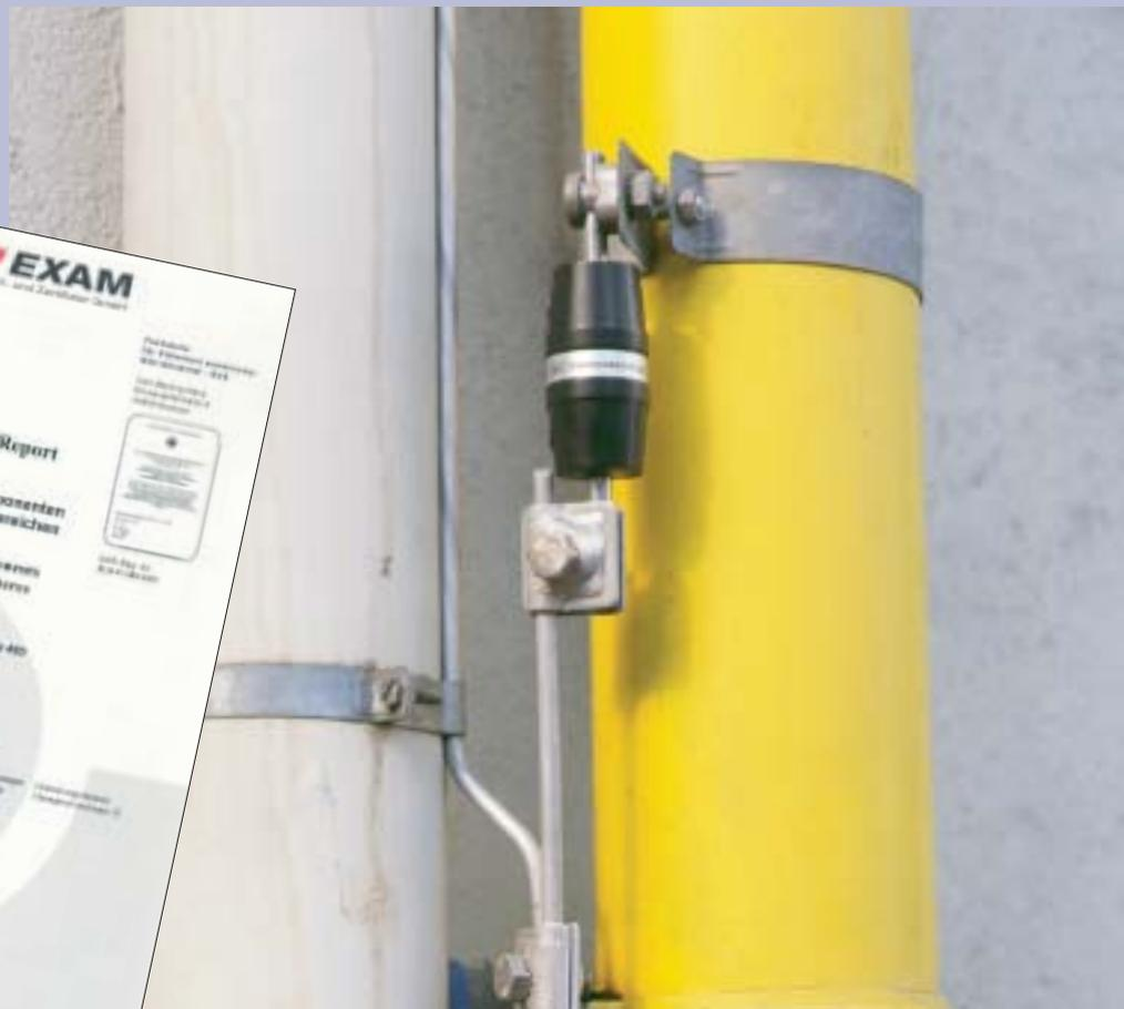
Fig.: Application example, isolating spark gap type 481
