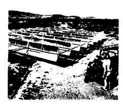
SOLAR THERMAL ELECTRIC research is being carried out on both large and small installations. Shown here is a 4 KW capacity array of concentrator collectors which heat a fluid that drives a turbine generator. The variable output of the array is fed into the AC service of the laboratory through a Gemini Synchronous Inverter. The future looks promising for solar thermal electric installations where insolation levels are high as is typical of the Southwest part of this country.
